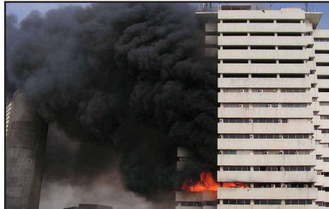
Building Fire Detection
