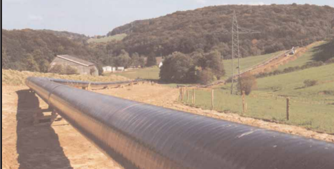
Oil and Gas Pipeline Monitoring
