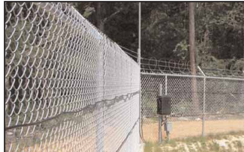
Border Security Monitoring
